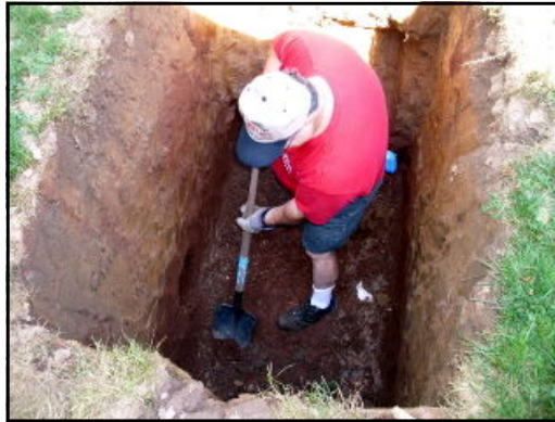
... and lots of work to make the hole ...
