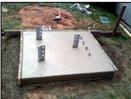
The base after the concrete pour on July 8th
